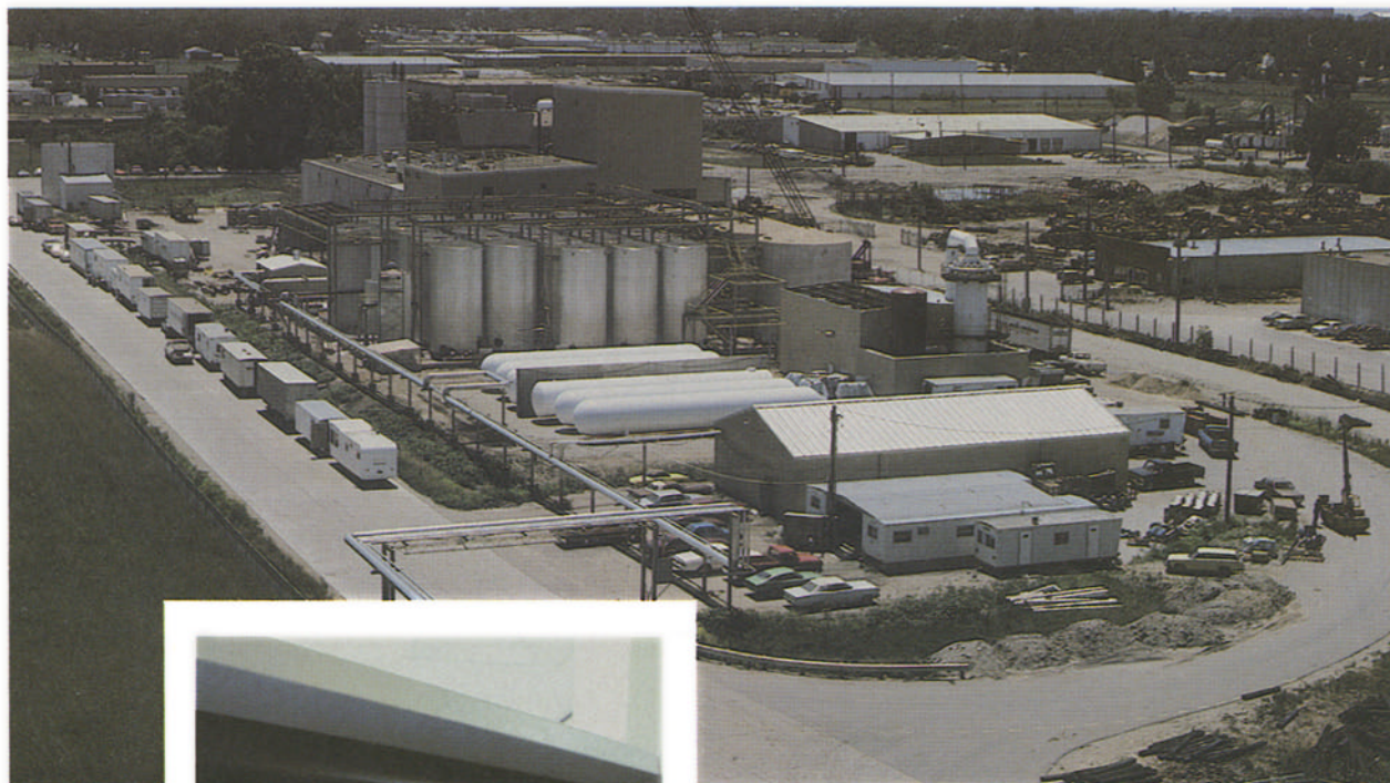
Staley refinery in Des Moines, Iowa
